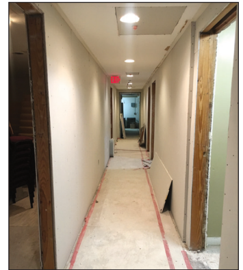
3rd Floor Hallway
